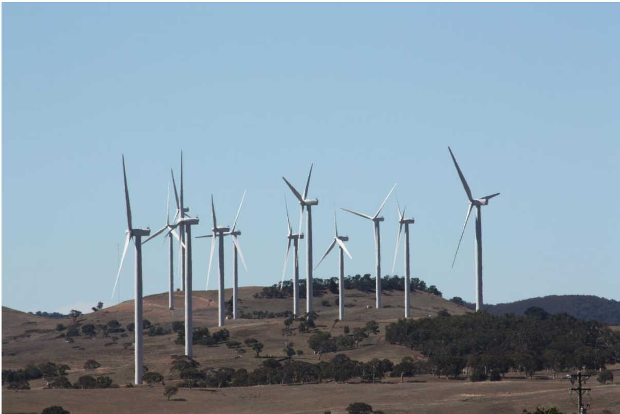
Windfarms near Canberra. Photo: ACT Government
